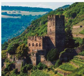
Gutenfels. Hotel. Kaub, Alemania. Aquarea y Aquarea Smart Cloud.
